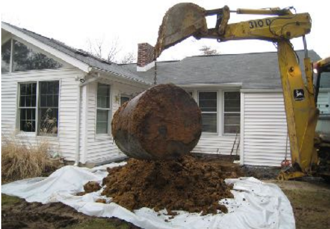
An old underground fuel tank being removed from a home in Wilmington
